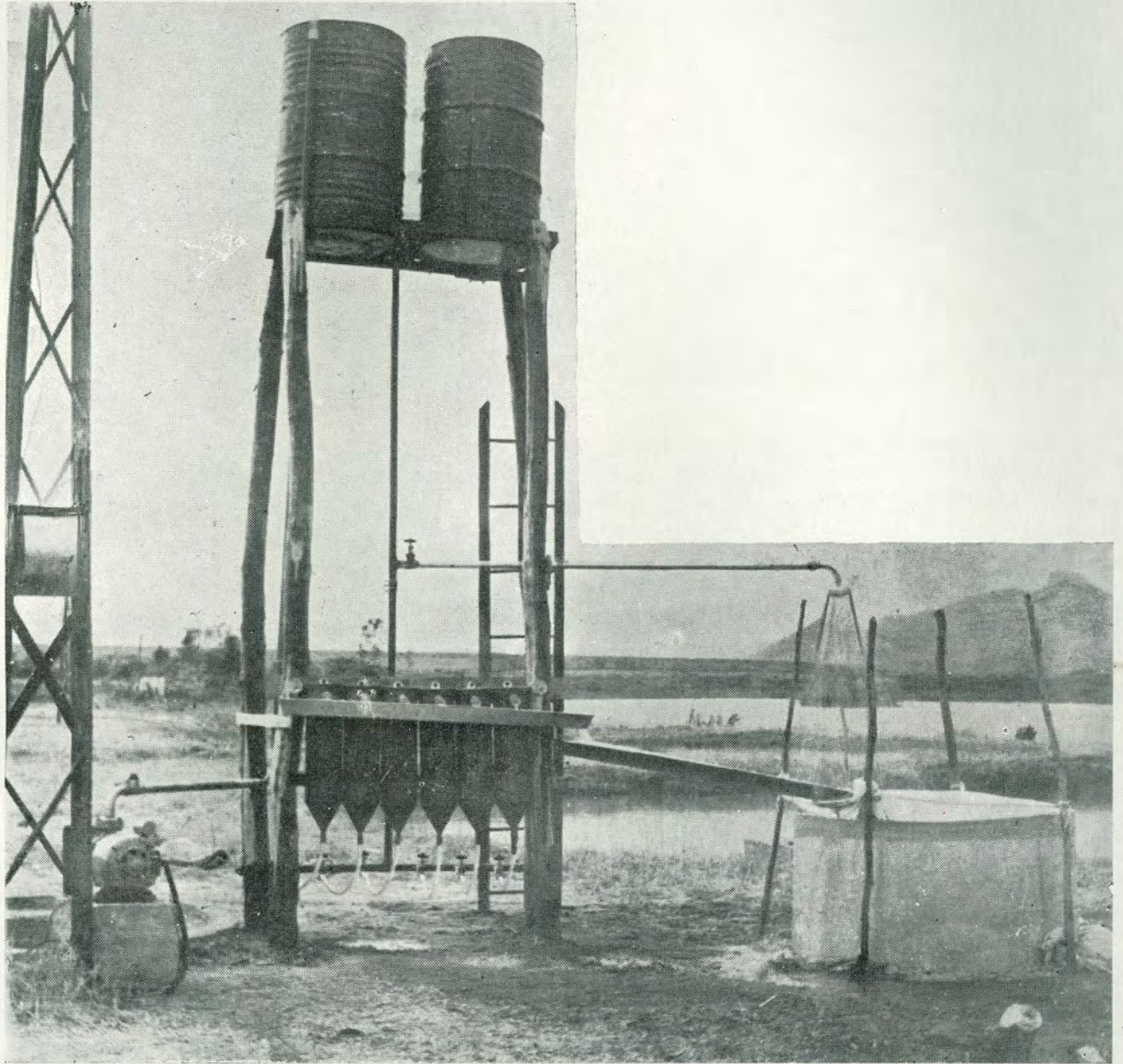
Field hatchery developed at CIFRI and installed at the Poongar farm at Bhavanisagar ( Tamil Nadu )
