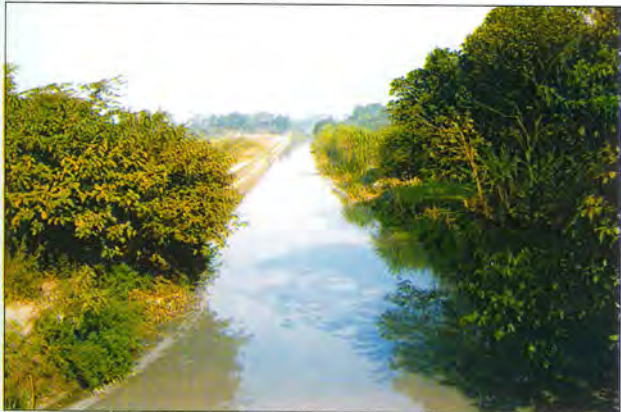
The flowing of effluent through cemented canal from thermal and steel power plant at Durgapur.
