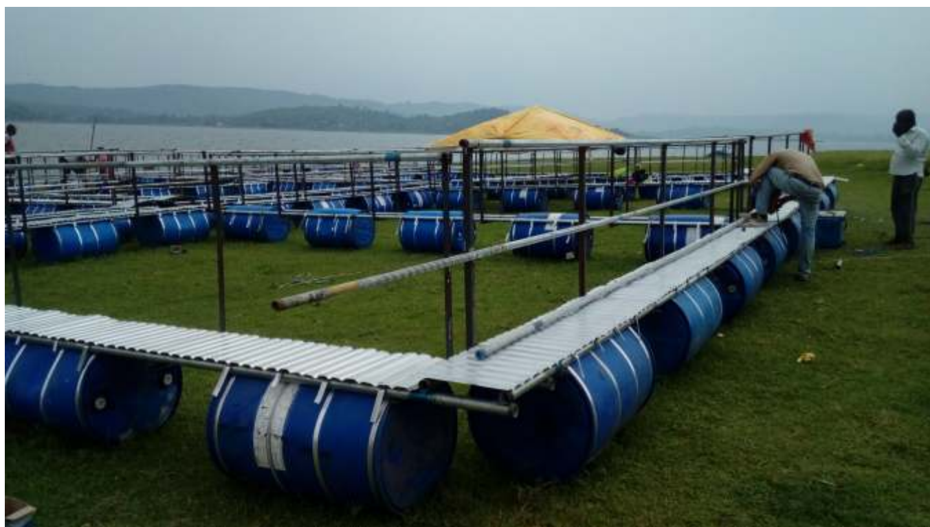
Fig. 149 Bird's eye view of CIFRI GI-Cage under fabrication
