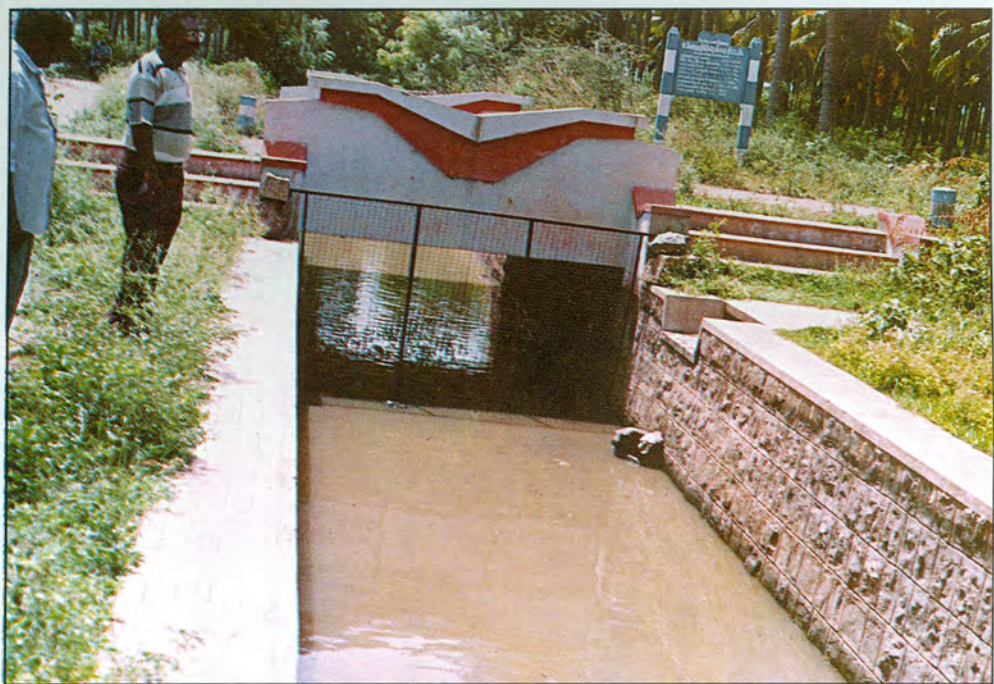
Weld mesh screen placed in the irrigation canal for preventing escapement of fish
