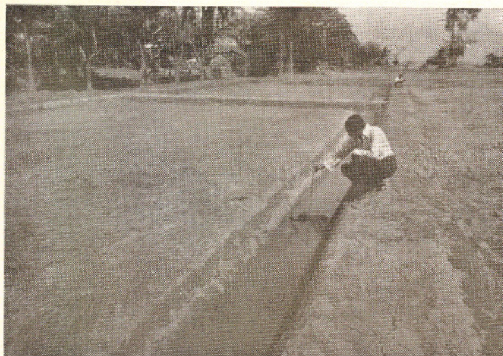
Plots are renovated by constructing dykes and digging perimeter canals.
